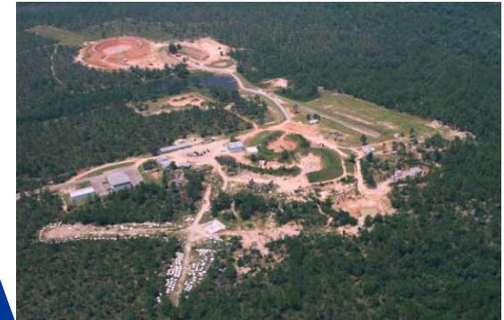
Rock Hill Facility DeFuniak, FL
